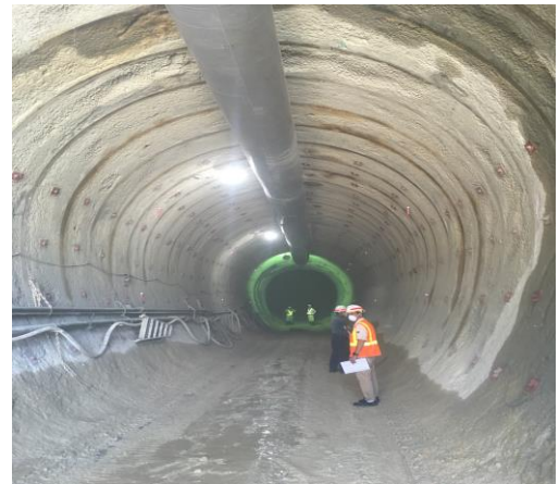
AGE Facility reroute diversion channel & tunneling project
